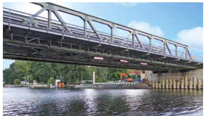
Freybrücke in Spandau
